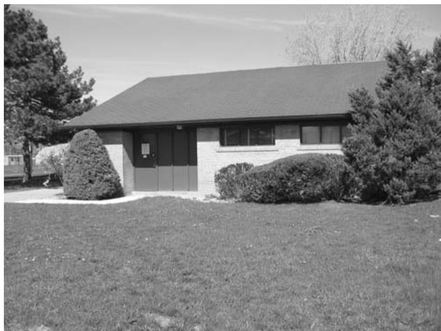
**Figure 9.3** A covert electrical substation.
